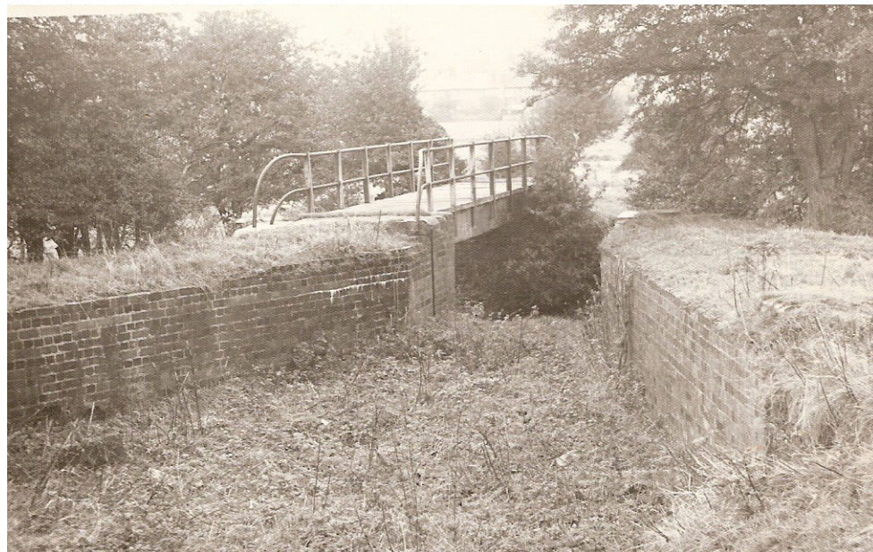
Entrance to the Aqueduct from the Basin (1968).
