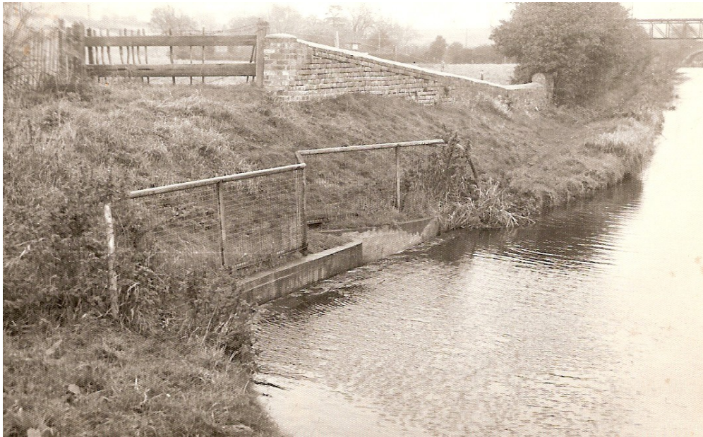
Entrance to the Stafford Branch Canal from the Staffs & Worcs Canal (1968).
